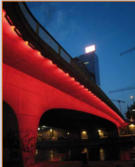
Vienna: Donaukanal bridge
